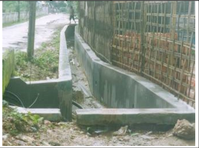
Construction of pucca drain at Girls' College Road, North Lakhimpur
