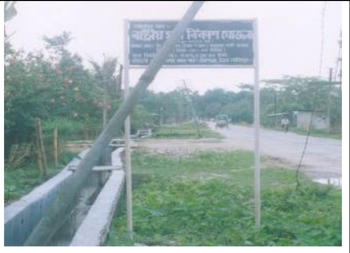
Construction of pucca drain along D.K. Road, N. Lakhimpur
