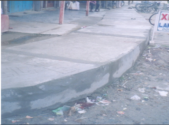
Construction of pucca drain at Bihpuria Sissapather Road
